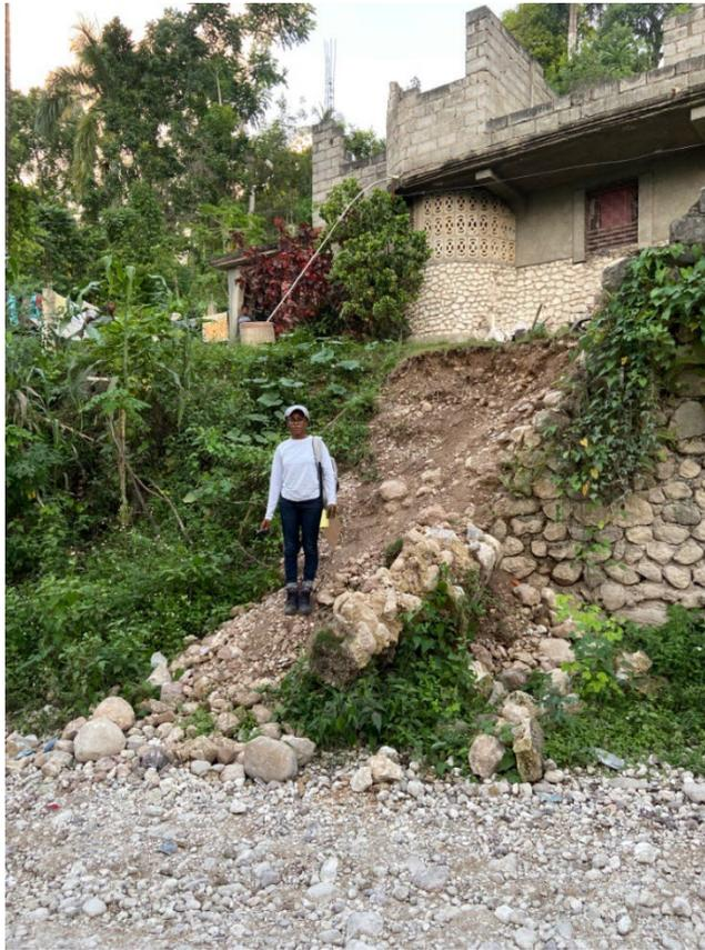
**Figure 7.102.** Retaining wall damage 2 km north of Enriquillo-Plaintain Garden Fault in Bonne Fin (Lat: 18.38944, Lon: -73.61028).
