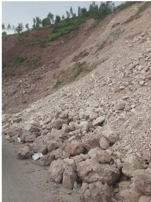
**Figure 7.30.** Rockfall along RN7 associated with 1.6 km stretch of landslide activity (Lat: 18.369867, Lon: -73.8784972). Photo taken September 27, 2021.
