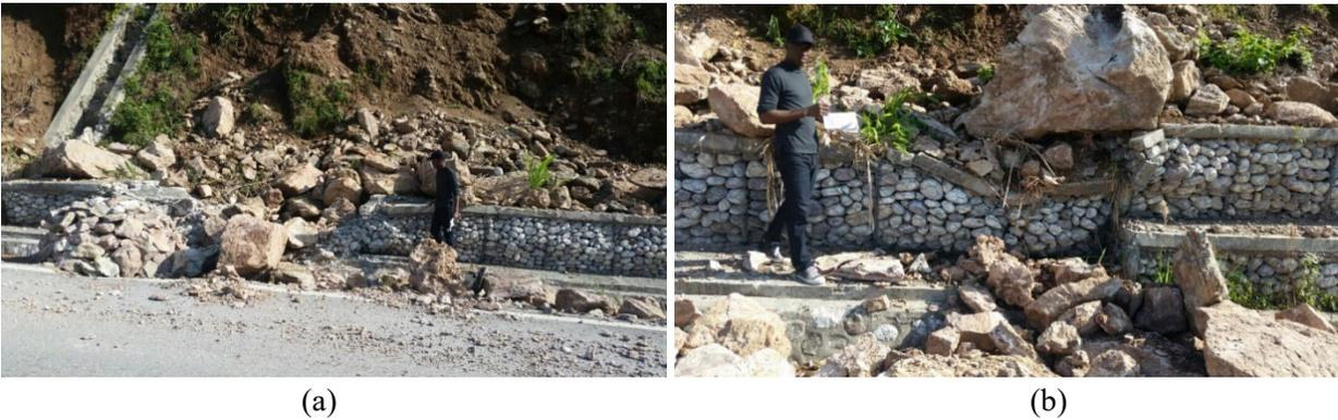
**Figure 7.99.** Retaining wall damage along RN7 (Lat: 18.403283, Lon: -73.8750032).
