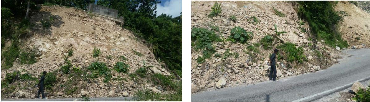
**Figure 7.26.** Slope failure along RN7 with water tank at top of slope (Lat: 18.3652708, Lon: -73.8791013).
