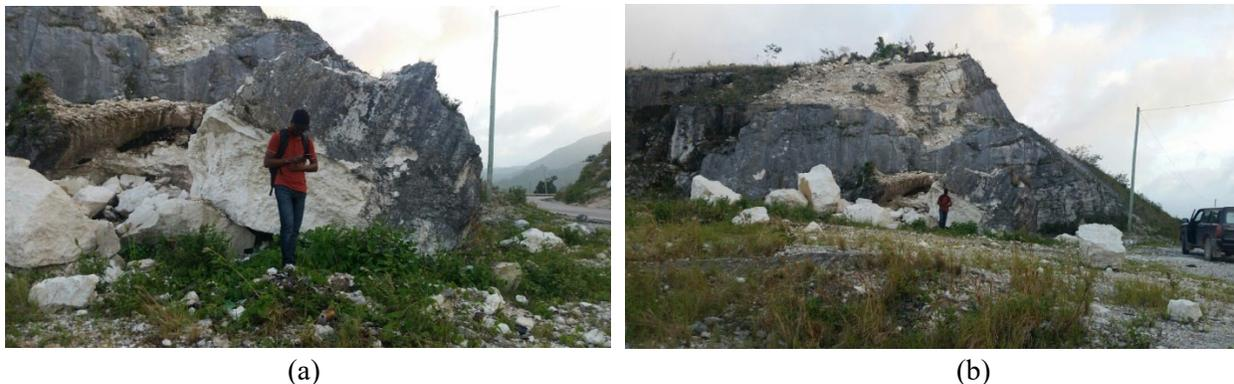
**Figure 7.58.** Possible failure of rockface along RN7 (Lat: 18.429466, Lon: -73.8998361).
